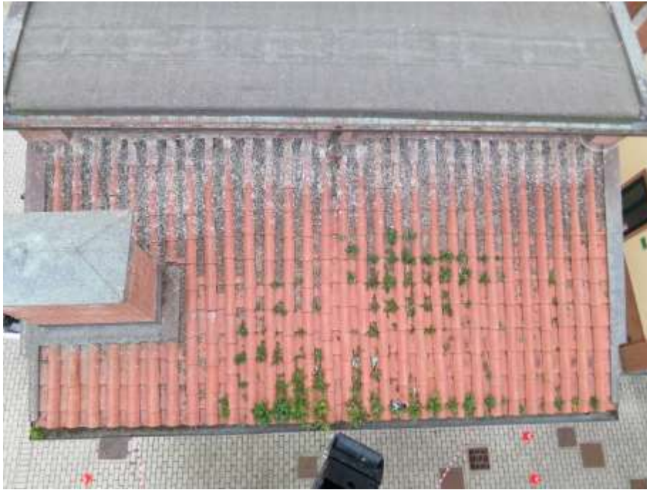
Figure 6. North roof prior to cleaning and treatment.
