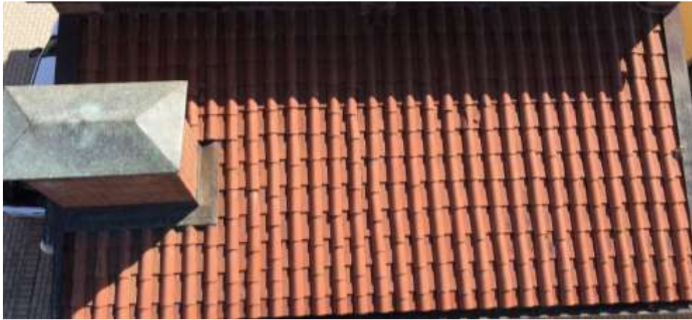
Figure 8. North roof after cleaning.
