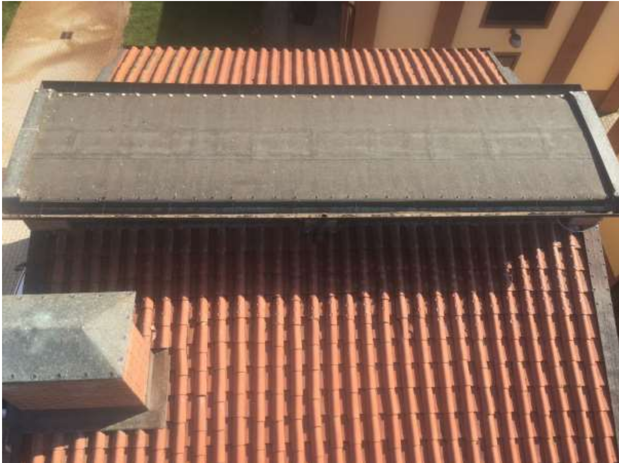
Figure 10. The area of the north roof treated with empty dishes was approximately 9m x 1.8m.
