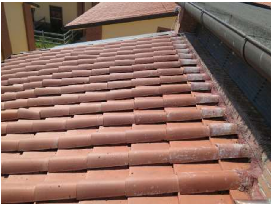
Figure 3. South roof after cleaning.
